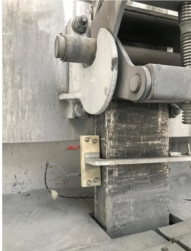
Figure 4. C-clamp installed on an anode rod.
